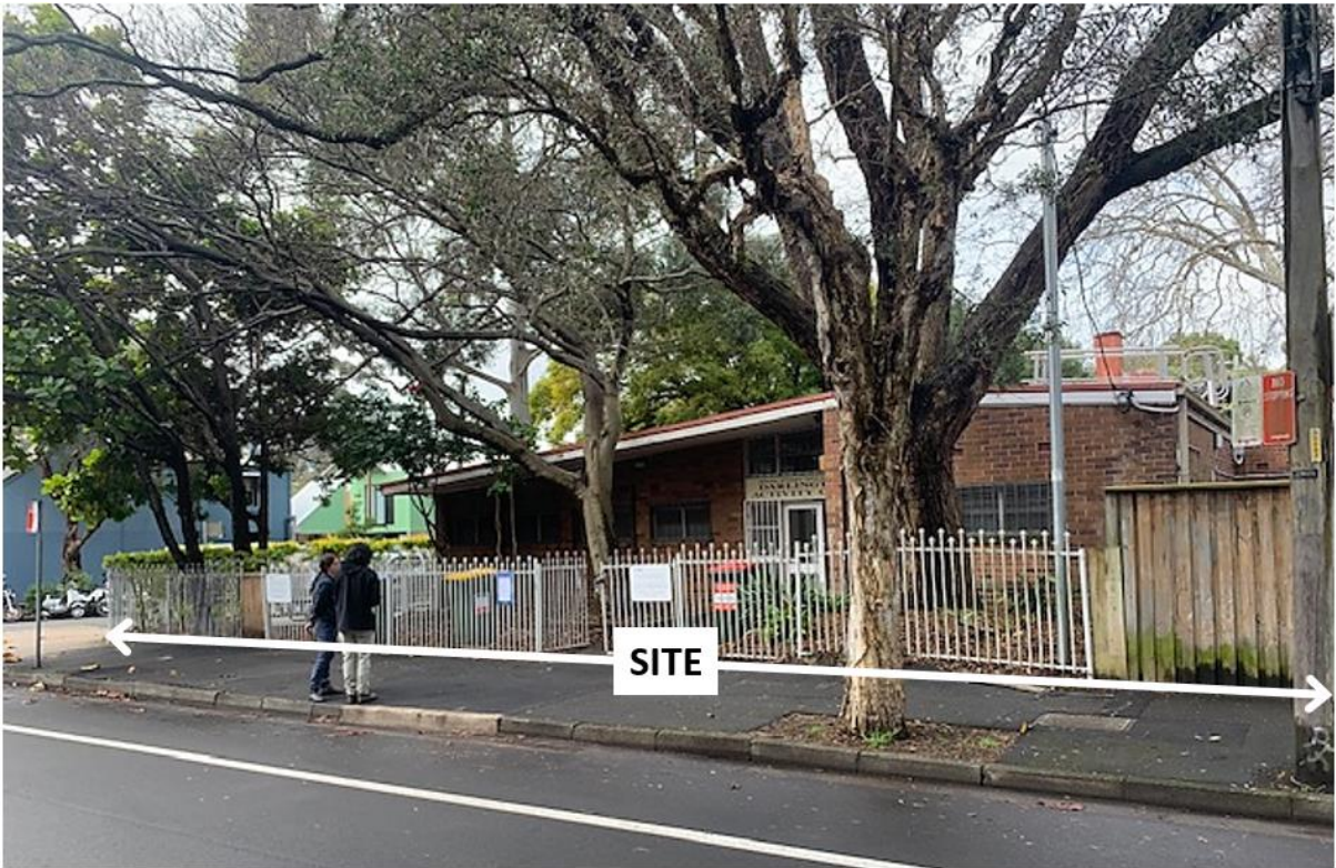
Figure 2: Shepherd Street (western) site frontage
